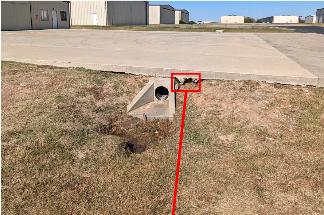
PHOTOS OF AIRCRAFT PARKING APRON TO RECEIVE FLOWABLE FILL – 10/19/22
