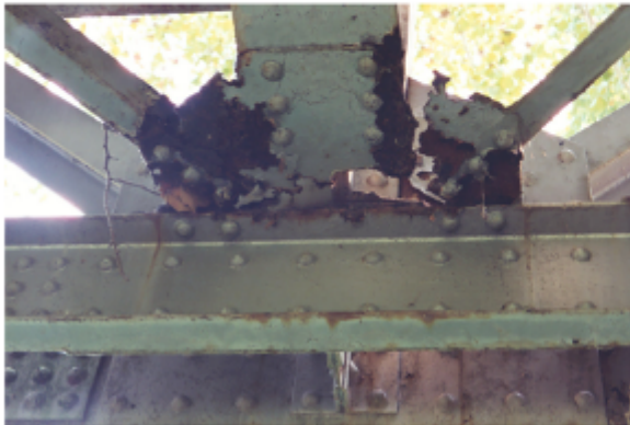
Corroded_Superstructure.jpg
