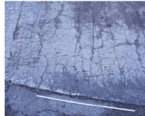
Deck Cracking 1.gif
