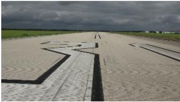
Figure 6. Runway 13-31, 31 End, Center.
