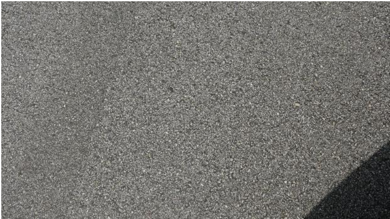
Figure 34. Apron A-35 Run Up, Close.
