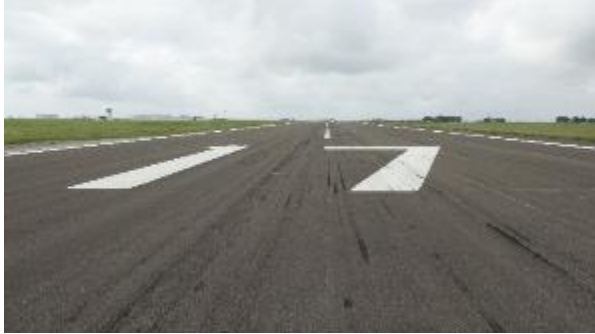
Figure 11. Runway 17-35, 17 End, Center.
