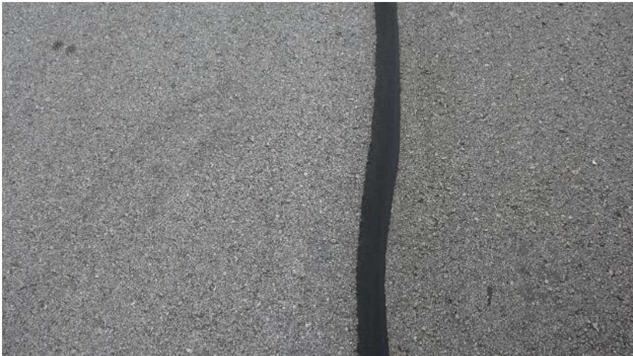
Figure 62. Taxiway T-F 31 A, Close.
