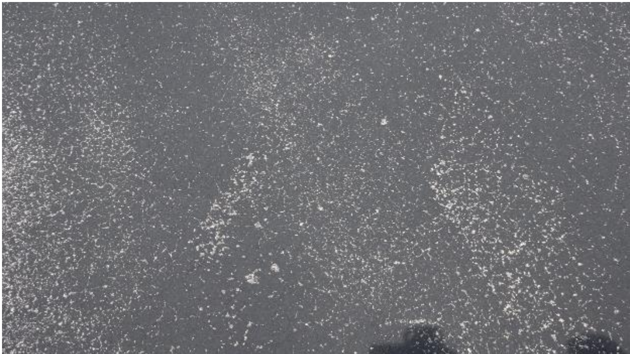
Figure 50. Apron A-T Hang A, Close.
