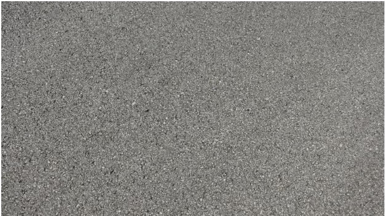
Figure 30. Apron A-31 Run Up, Close.
