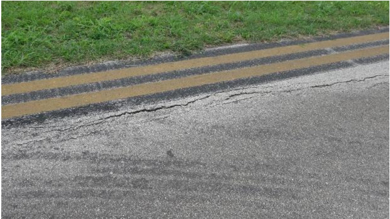
Figure 67. Taxiway, T-A C G. High Severity Crack.
