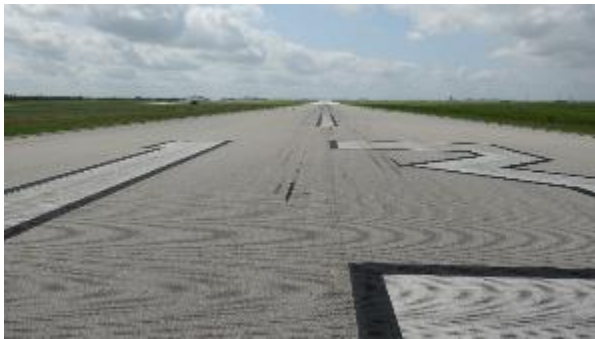
Figure 1. Runway 13-31, 13 End, Center.
