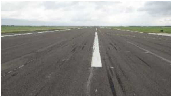
Figure 16. Runway 17-35, 35 End, Center.
