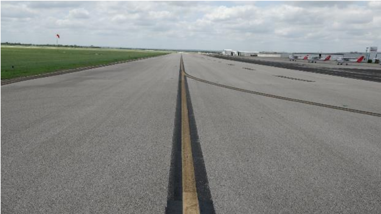
Figure 59. Taxiway T-A East.
