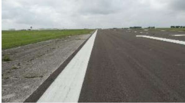
Figure 12. Runway 17-35, 17 End, Inside Edge.
