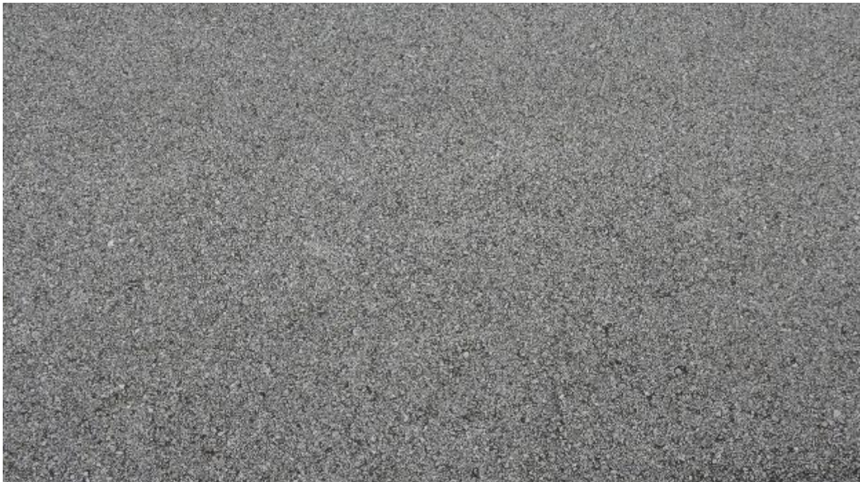
Figure 62. Taxiway T-G, Close.
