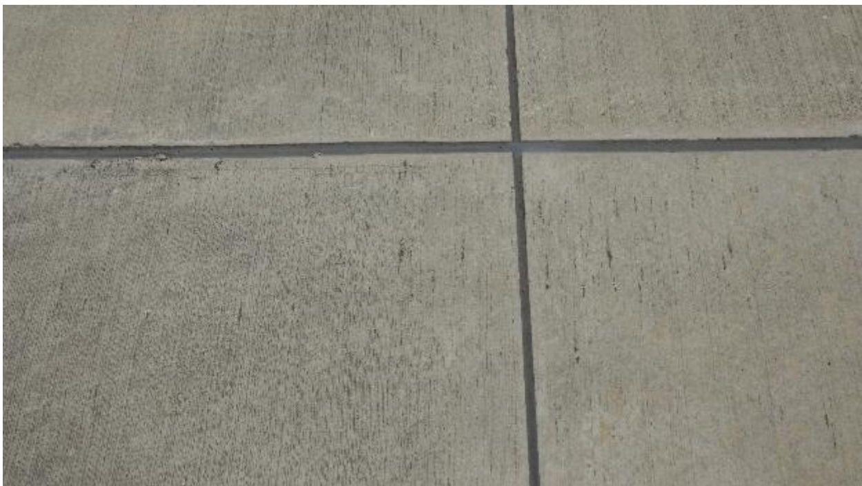
Figure 48. Apron A-PCC, Close.
