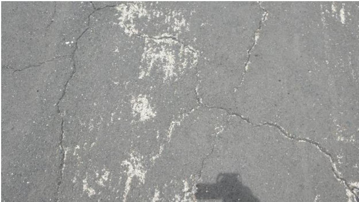
Figure 38. Apron A-East, Close.
