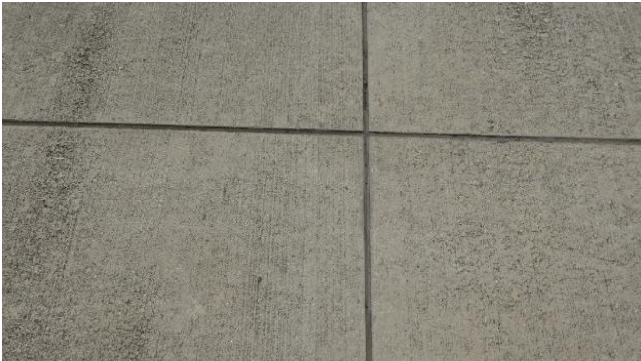
Figure 40. Apron A-Fuel, Close.
