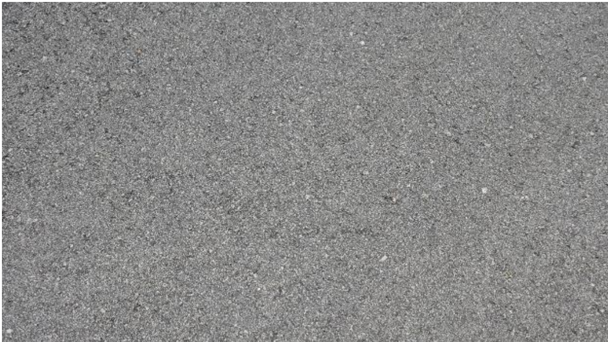
Figure 56. Taxiway T-A B C, Close.
