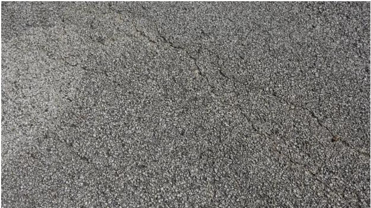
Figure 28. Apron A-2317, Close.
