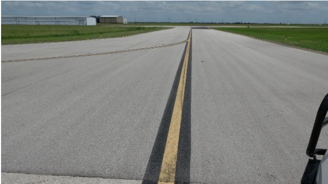
Figure 61. Taxiway T-A F G.
