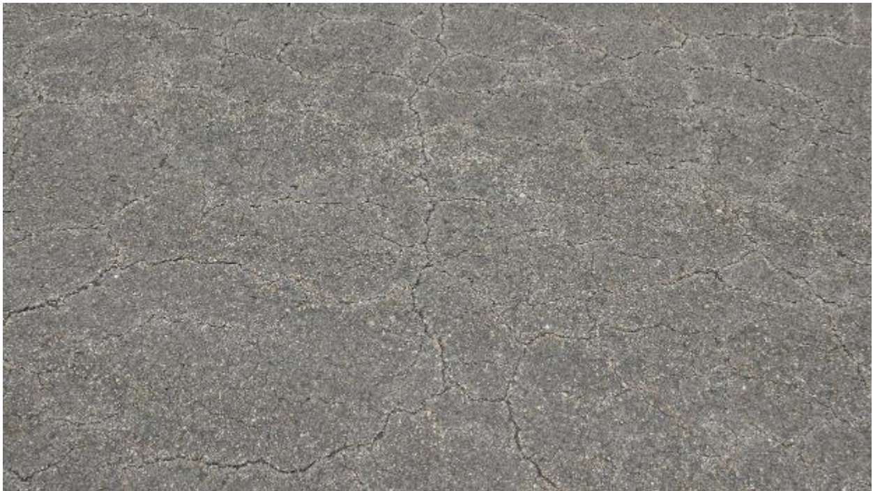
Figure 22. Apron A-1756, Close.
