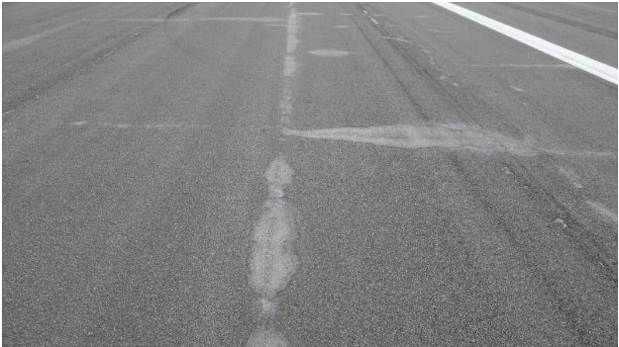
Figure 66. RW 17-35. Pumping Cracks
