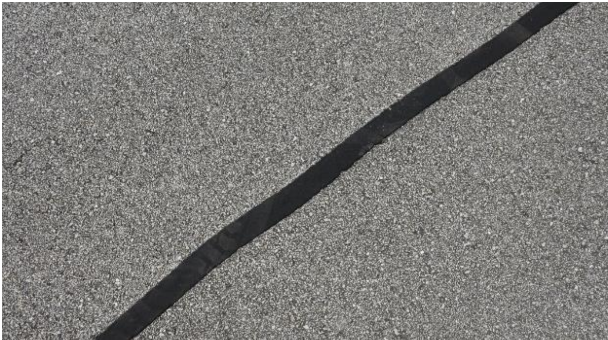
Figure 62. Taxiway T-F, Close.
