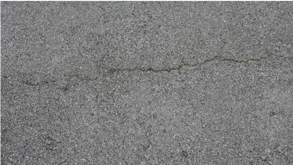
Figure 60. Taxiway T-A East, Close.
