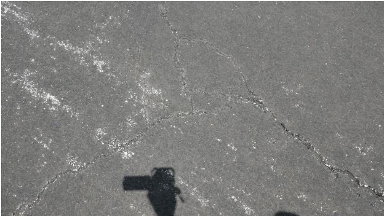
Figure 26. Apron A-1806, Close.
