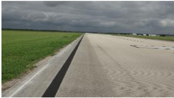
Figure 7. Runway 13-31, 31 End, Inside Edge.
