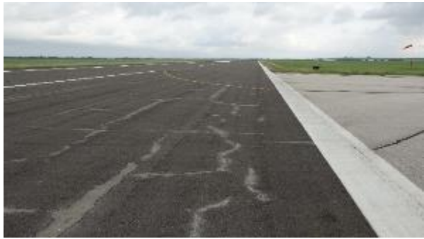
Figure 17. Runway 17-35, 35 End, Inside Edge.
