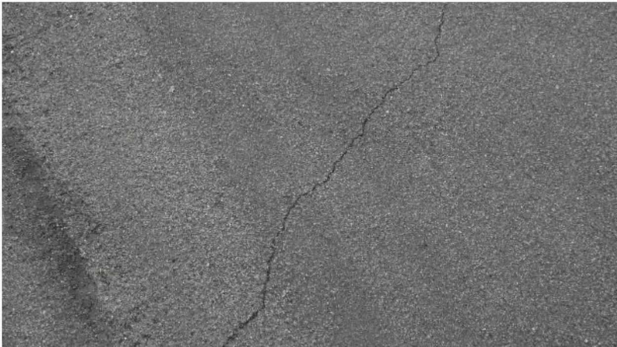
Figure 32. Apron A-35, Close.
