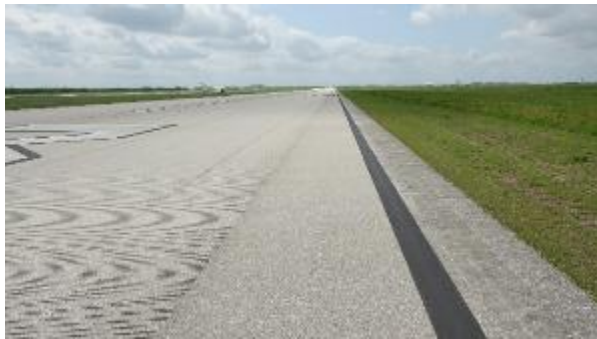
Figure 2. Runway 13-31, 13 End, Inside Edge.
