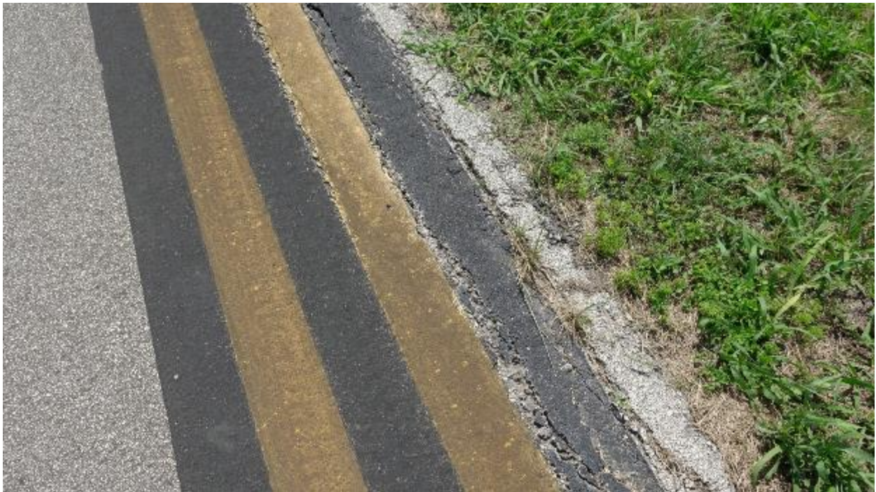
Figure 68. Taxiway, T-E East. Edge Damage
