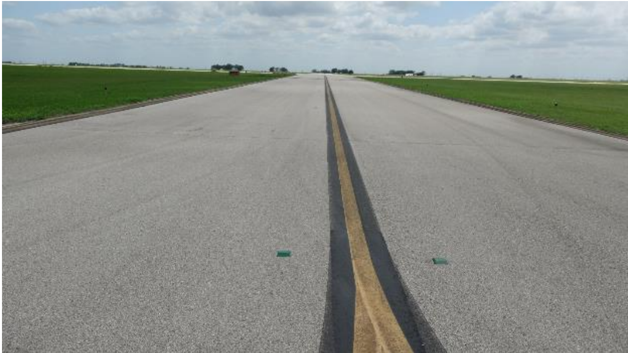
Figure 61. Taxiway T-E East.
